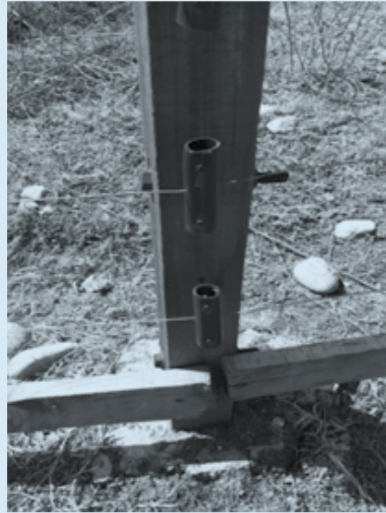
Fig. 6 & 7: The noticeable difference in the life span of the post fixed on the iron clamp and one set in the soil.
