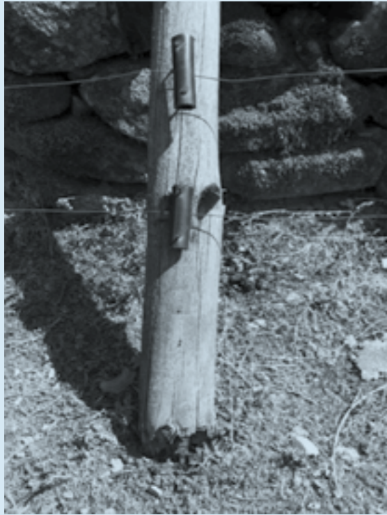
Fig. 6 & 7: The noticeable difference in the life span of the post fixed on the iron clamp and one set in the soil.
