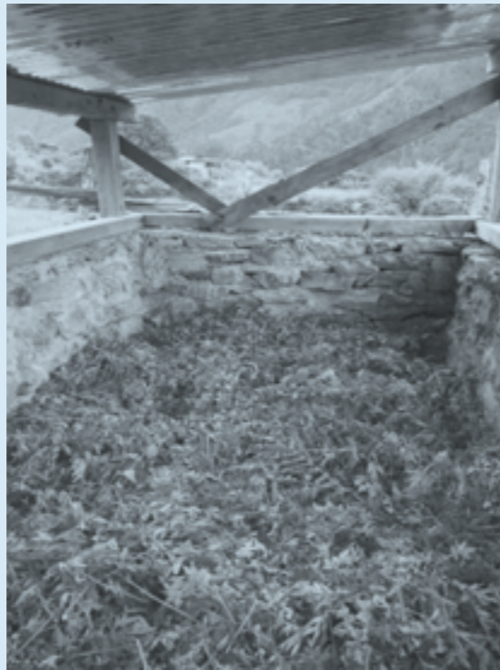
Fig. 13 & 14: Heap composting and compost shed at Engo Village.
